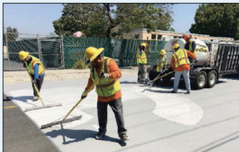
Photo 5: Applying cool pavement coating
