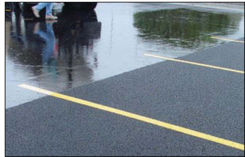
Photo 9: Porous asphalt allowing water to infiltrate next to an impermeable pavement
