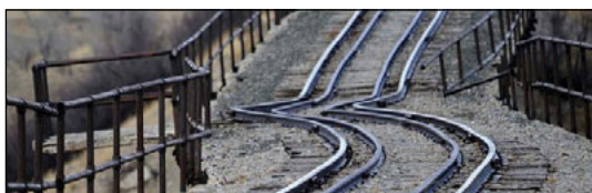
Photo 1: Rails buckled due to heat
